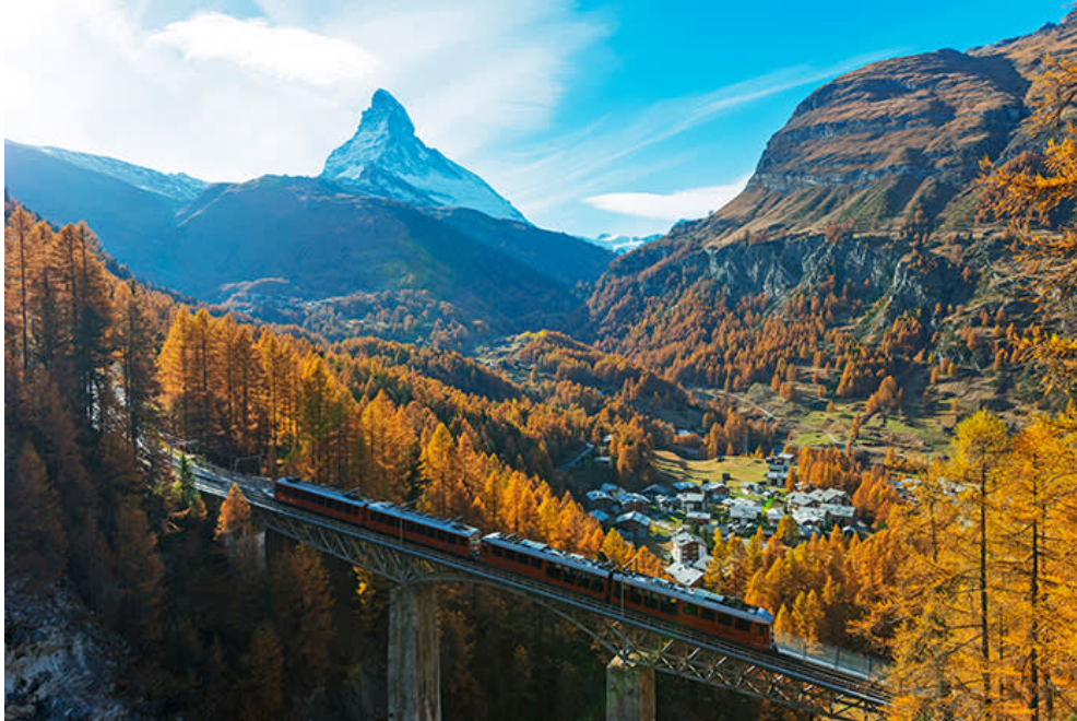
The Glacier Express traverses Findelbach bridge in the Swiss Alps © Christian Kober
