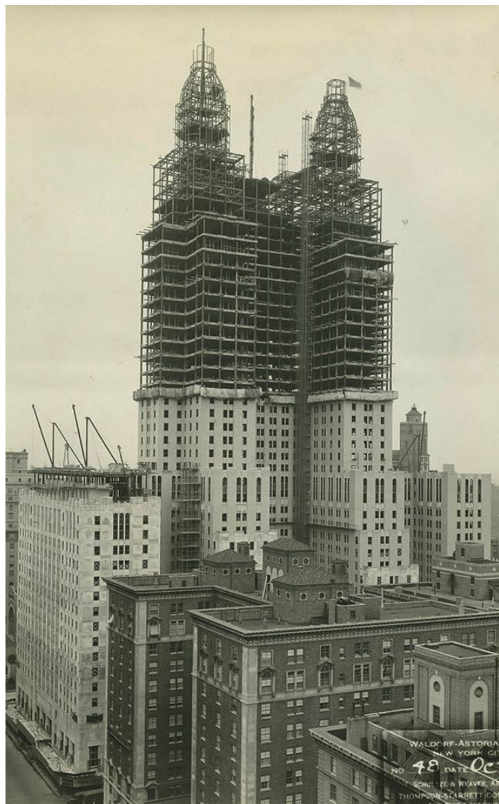
Waldorf Astoria under construction, 1930
