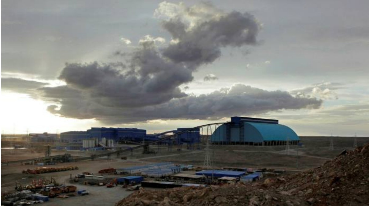
The underground expansion of the Oyu Tolgoi mine has been beset by problems © REUTERS
